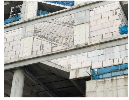
Typical AAC wall using regular blocks and jumbo blocks, external and common areas.
