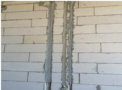
AAC wall with concealed M&E services.
