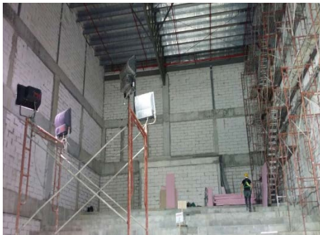
AAC wall with columns.
