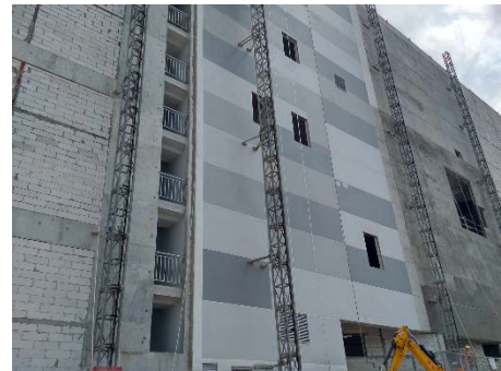
AAC wall, externally applied with plastering and paint.
