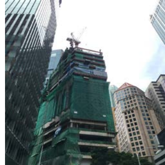
ROBINSON TOWER (Robinson Road)
