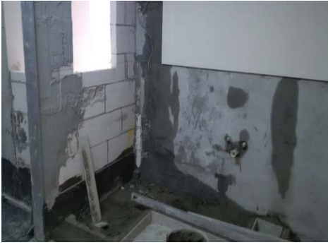
AAC wall in wet area with waterproofing and services pipes.
