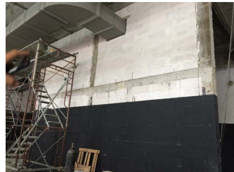
AAC wall with large M&E items. Lintel provided in openings.
